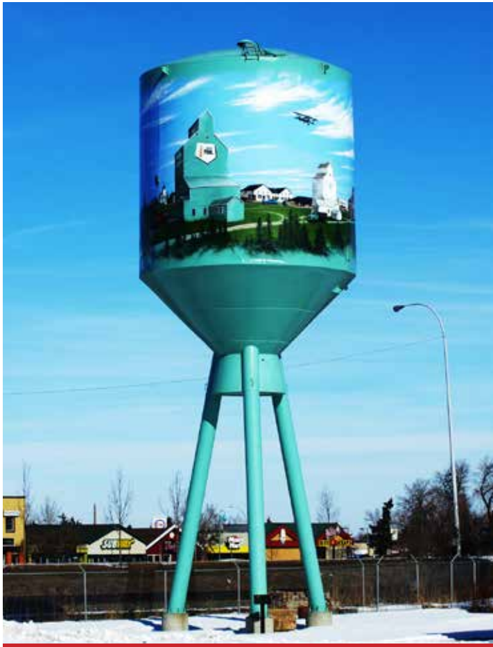
Left: The restored water tower at Spruce Grove, Alberta, was rescued after it had been dumped in a farmer's field and abandoned for years. Right: This unique lighthouse-style water tower in Humboldt is one of only four left in Saskatchewan. Once slated for demolition, the century old tower is now a popular attraction.
