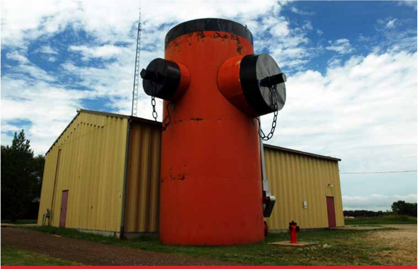
The fire hydrant tower at Elm Creek, Manitoba, was built to be a water source in 2001 by volunteer firefighters and is arguably the largest of its kind in the world.
