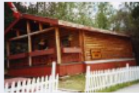
Eight Avenue Dawson City YT
