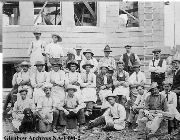
Public library under construction, Calgary, Alberta.
