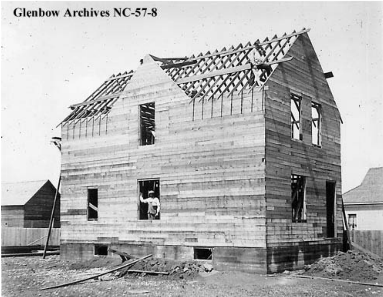
Clipsham house under construction, Calgary, Alberta. ca. 1911-1912
