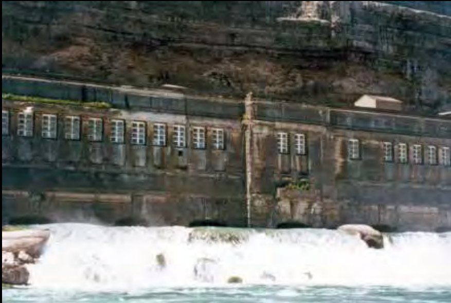
Power House of the Electrical Development Co. of Ontario, Ltd. Operated by The Toronto Power Co., Ltd., Niagara Falls, Ont., Canada
