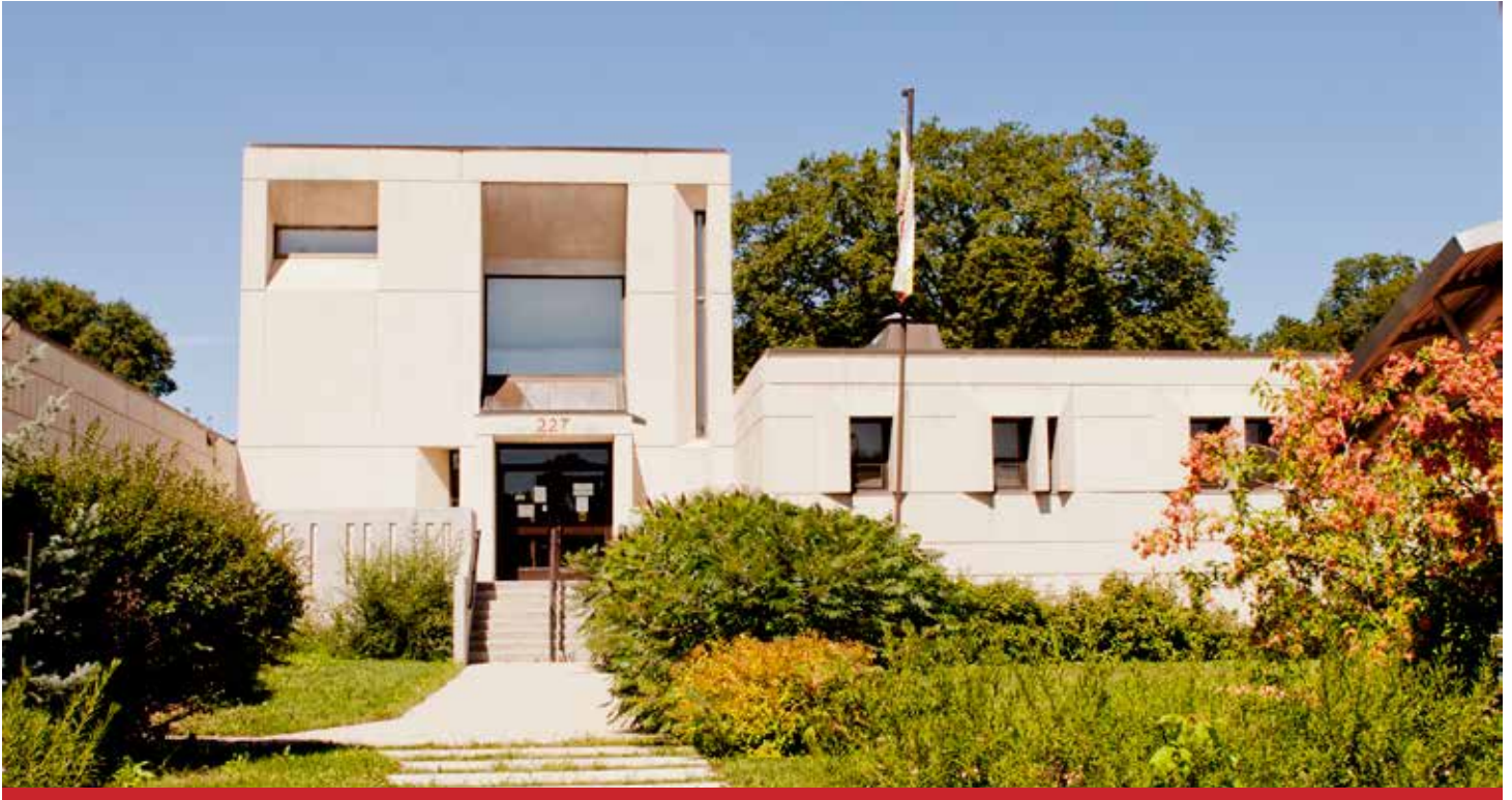
St. Boniface Civic Centre (1964) consists of three buildings designed in a Brutalist institutional style set around a park-like plaza. Defining elements include pre-cast stone veneers with vertical patterning, deeply inset windows and doors, and heavy masonry mullions. (Designed by Étienne Gaboury.)
