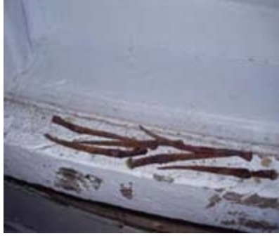
Original forged siding nails. The nails had corroded in the siding area, but remained sound where they were nailed into the framing.
