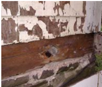
Evidence of failed paint can be seen on the rear wall shingles.
